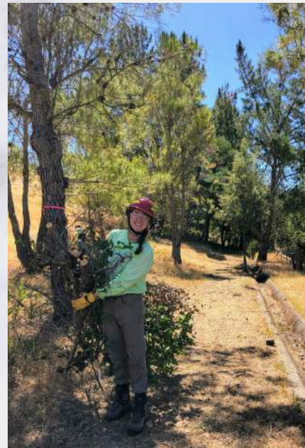
Elise Oswald removes vegetation along a fireroad.
