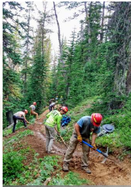
Trail maintenance near Curly Lake
