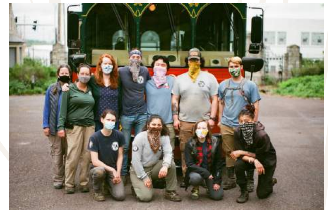
During a trail construction project at Bellefontaine Cemetery & Arboretum, Members served with Dee Van Huss (2nd from left), Year 18-21, Bellefontaine's Horticulturalist.
